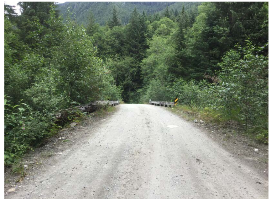
Approach from Left Bank when facing downstream
