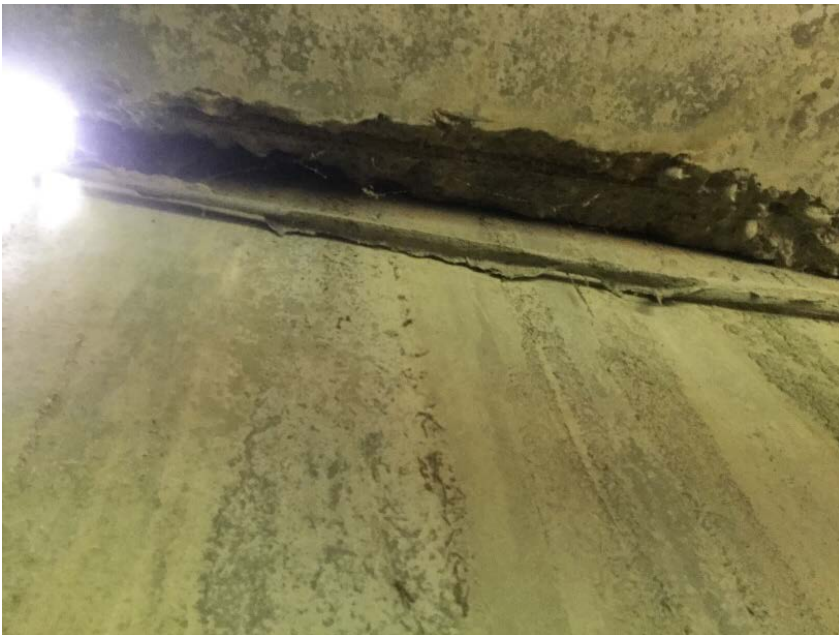
Right bank, panel 1 from underneath
