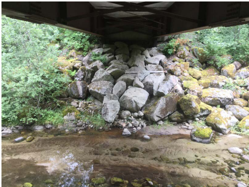
Right Bank Abutment when facing downstream
