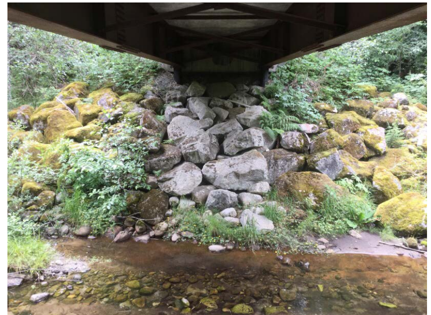
Left Bank Abutment when facing downstream
